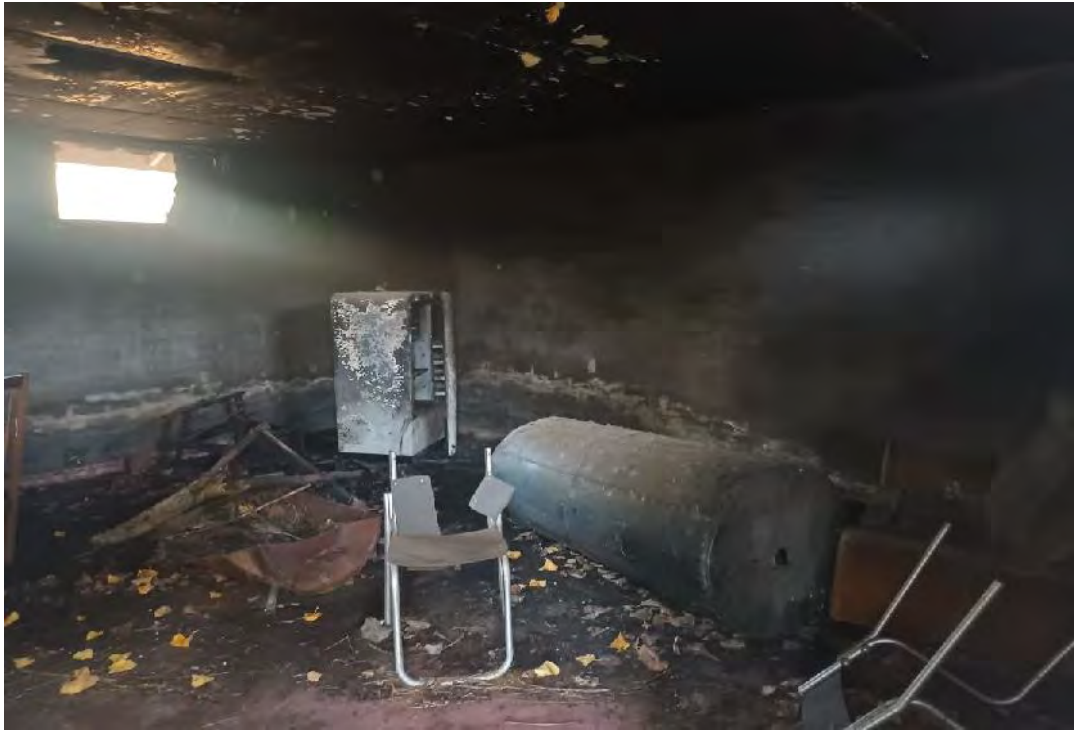
Photo 8: View of burnt interior and contents within fire fighting training structure.
